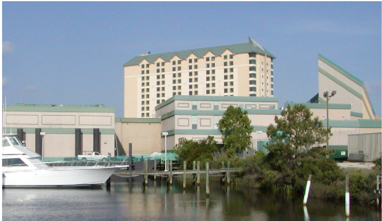
(Above) View of Hotel from West
