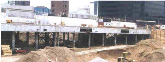
Lawrence Street Under Construction
